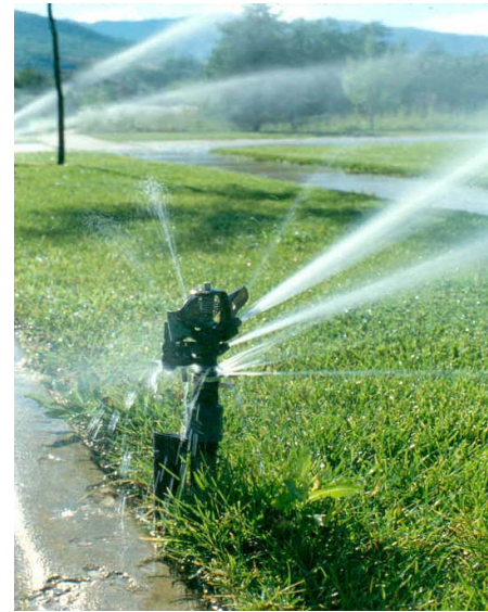
Watering at wrong time of day
